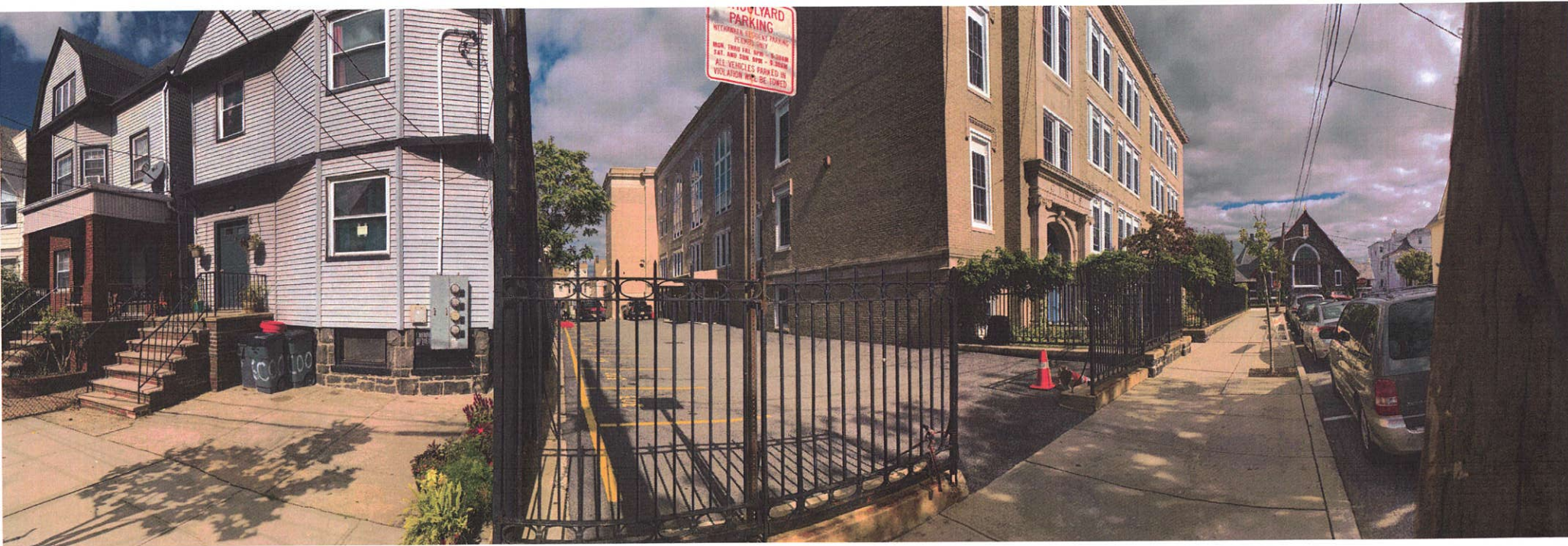
Photo 5: (Panoramic Full View: EXISTING Front Right Side Yard & Adjacent to School) PROPOSED: Location of Proposed Brick-Paved Driveway and New Flower Box Right Side Landscaping Improvement.
